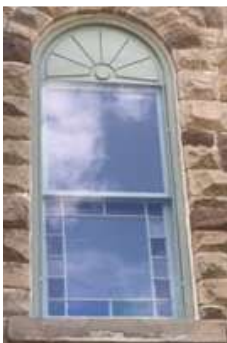
New storm windows
